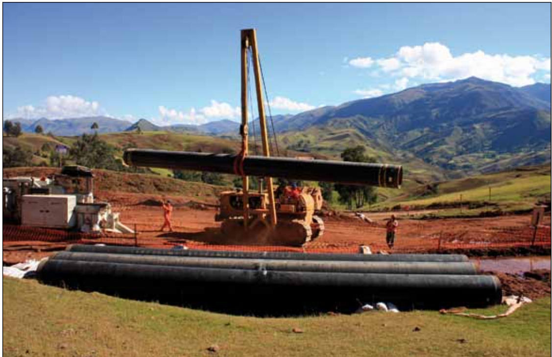
Laying the pipeline to supply Pampa Melchorita.
